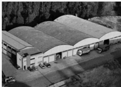
Expansion of a new 1000m 2 building
