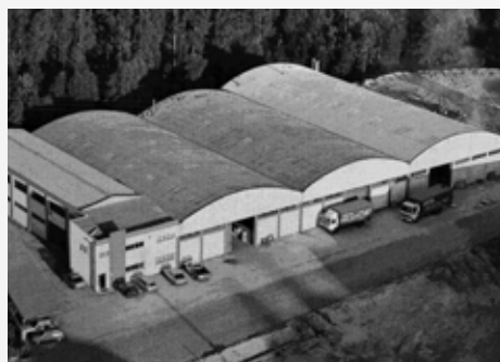
Expansion of a new 1000m 2 building
