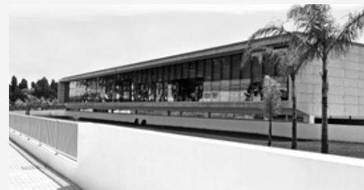
Construction of the new 17.000 m 2 factory
